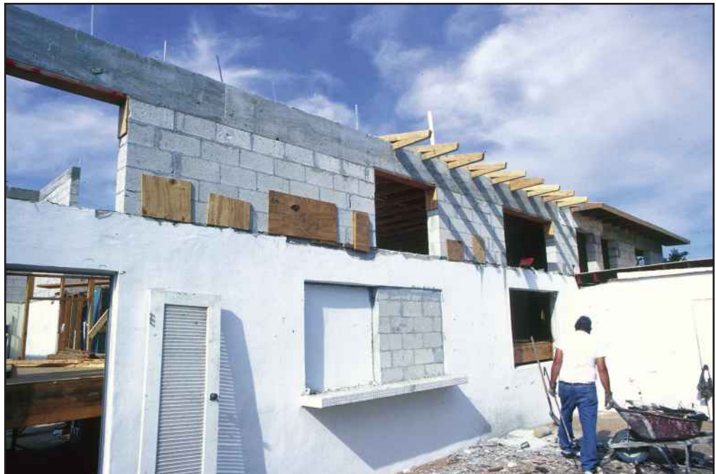
Figure 67 The extended first-story walls.
